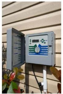
WaterSense labeled Irrigation Controller
